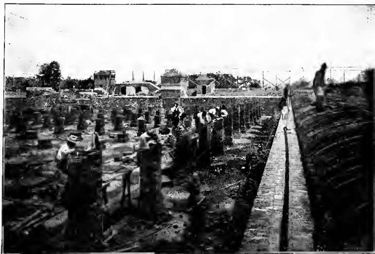
BUILDING THE BRICK PIERS.
